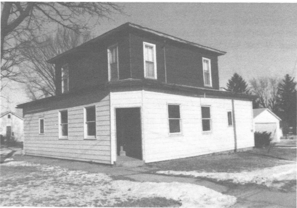
S. 4th & Collins Railroad Hotel and Restaurant. Run for many years by a Mrs. Lester. Later by the Orvil Hiscox, Sr. It was built when the railroad came across the river. Present owner: Francis Saunders. (Photo by Donna Kennedy).
