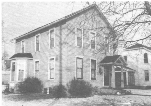
210 S. 6th St. Original owner: Prentice R. T.—Purchased by Frank Zeigler in early 1930s. Part was moved to 108 S. 6th St. Both houses were remodeled at that time. Present owner of 110: Joyce Thompson. Present owners of 108: John C. and Judy Zeigler. (Photo by Donna Kennedy).
