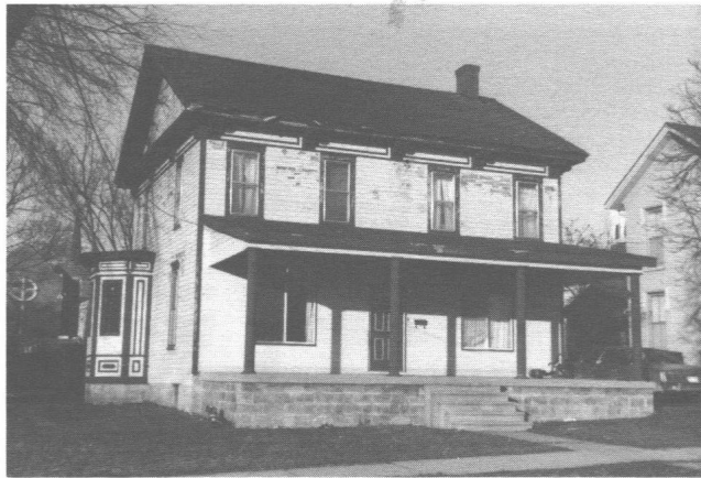
202 South 3rd St. Builder not known. 1905 residence George H. Jones. Other owners: Harry Harnish, Levitt and Mary Jones. Present owner: Robert Nielson. (Photo by Donna Kennedy).
