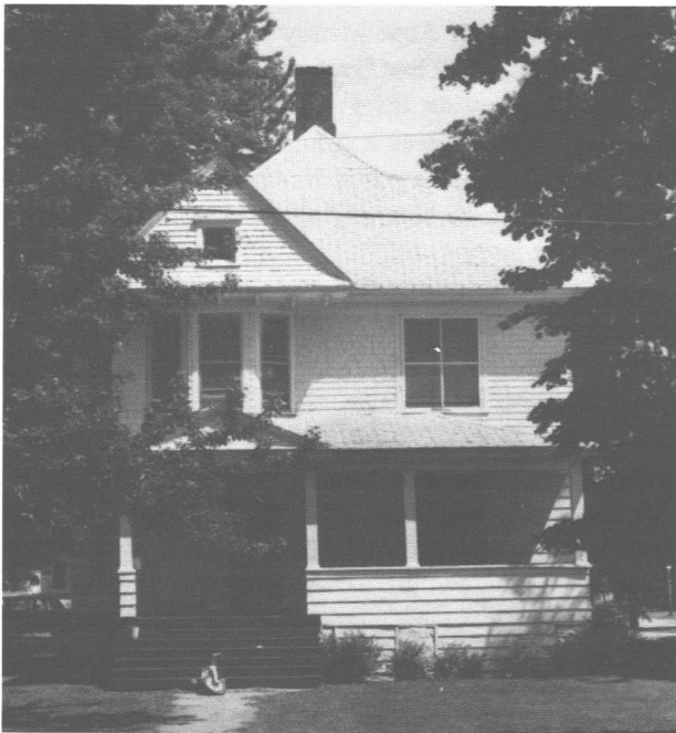
500 North Fifth Street Owner in 1898 was Frank E. Reed, Attorney, who in the early 1900's was an Ogle County Judge. During the middle 1900's this property was made into apartments and was a rental property. Present owner is Robert Adamson. (Photo by Donna Kennedy)
