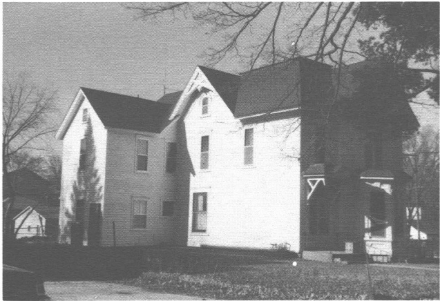
300 South 3rd Owner in 1898 was Calvin J. Seyster, rented later as an apartment house. Present owner James Lauer. (Photo by Donna Kennedy).
