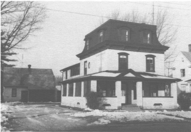
402 S. 4th St. Fredrick G. Petrie-original owner. Purchased three lots in 1863. Petrie was one of the owners of the east side Grist Mill. This home was built in the 1860's. The unusual style of roof is called a Mansared (French type of roof, popular in the U.S. from 1860 to 1880). Since 1965 owners: Charles F. Anderson purchased in 1925, and started the Oregon Dairy. Carl Anderson, his son, continued the dairy. Frank Fischer in 1939. Present owner: Mrs. Fredric G. Deuth. (Photo by Donna Kennedy).
