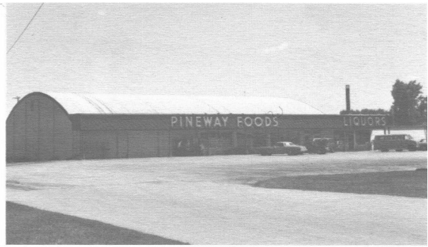
Pineway Foods and Liquors. Tenth Street and Pines Road. Dan Durl
