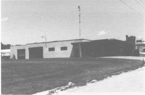
C. H. Ehmen Industries. Heating-Plumbing. Route 64 East. Gary Fruin
