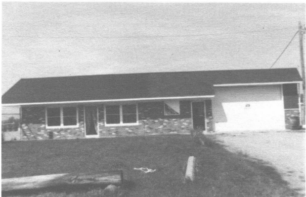
Commonwealth Edison. Daysville Road.
