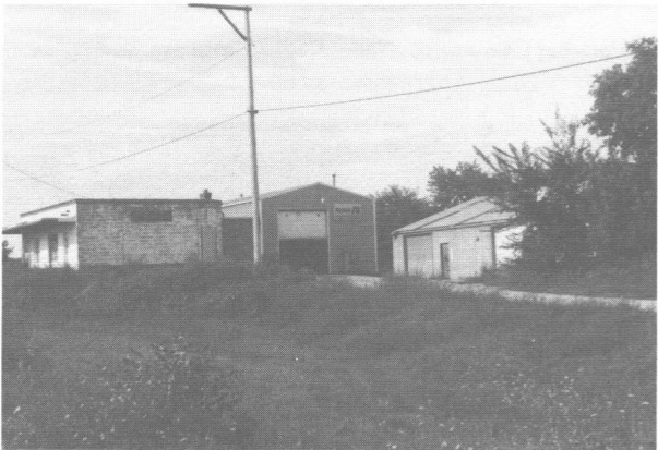
Ruan. West side of viaduct on Highway 2, South.
