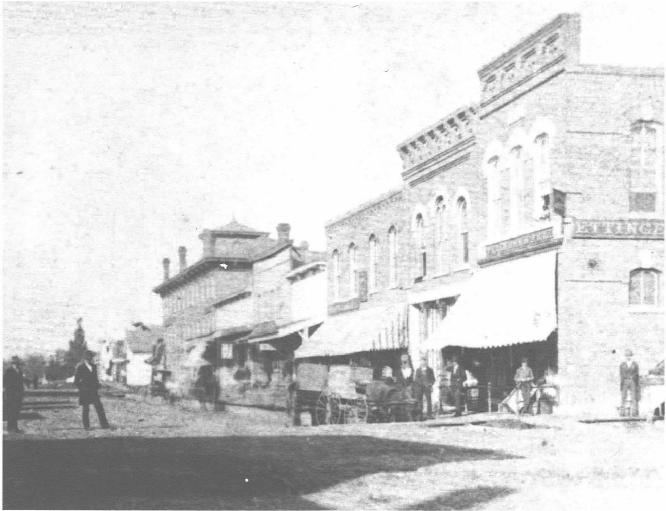
300 block of Washington Street (north side)
