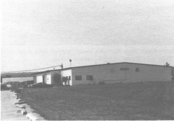
Atwood Vacuum Machine Company. Pines Road. Steve Korth.
