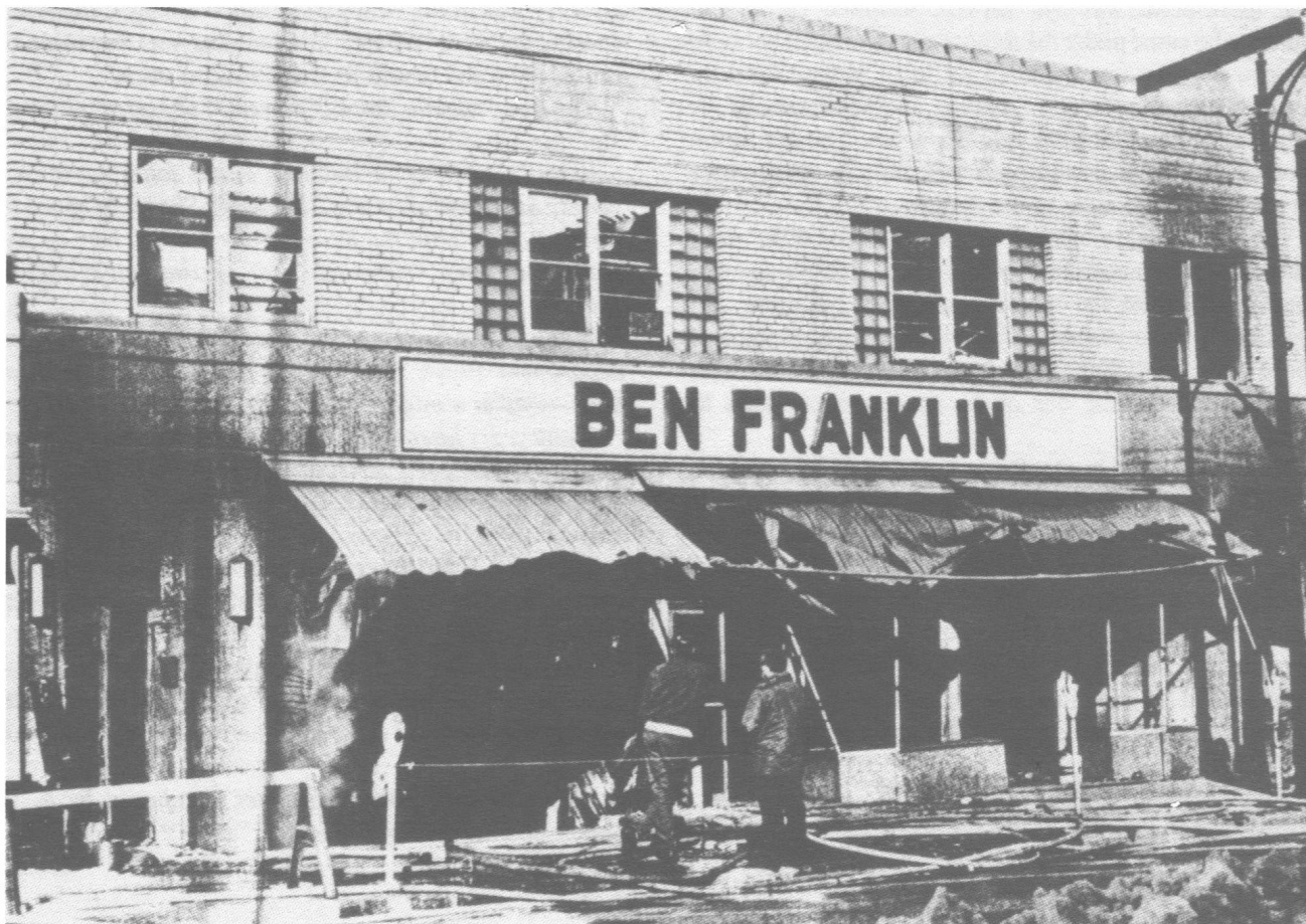
A tragic fire which began in the Hawk Bowl, gutted the bowling alley, the Ben Franklin Store, and the second floor apartments.
