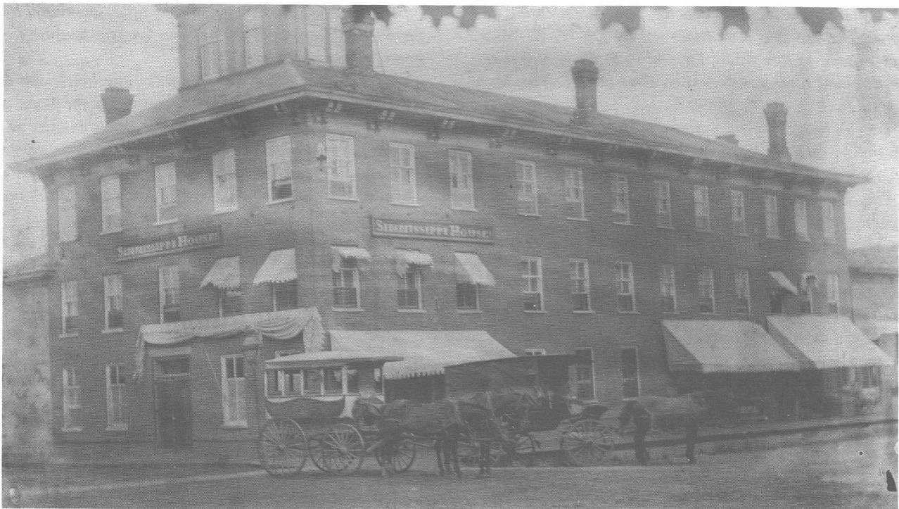
Sinnissippi House before the turn of the century and name changed to Sinnissippi Hotel. Built in 1847. This picture is from 1890-1900—wagon in front was used to transport guests to depot. Heated with stoves instead of a boiler. Addition at left-hand corner was torn off later. Barber shop and variety store may have been under awnings at right-hand side of picture. (Photo courtesy of Republican Reporter)
