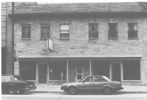
121-123 South Fourth Street Fischers Book Store (N. half); then Clifford and Bryson (toy makers) (all of building); then Piggley Wiggley; then Charles Lamb Firestone Store; the Oregon Home Appliance 'til 1981; then Deuth and Reising Insurance as remodeled in 1947. (Photo by Donna Kennedy)
