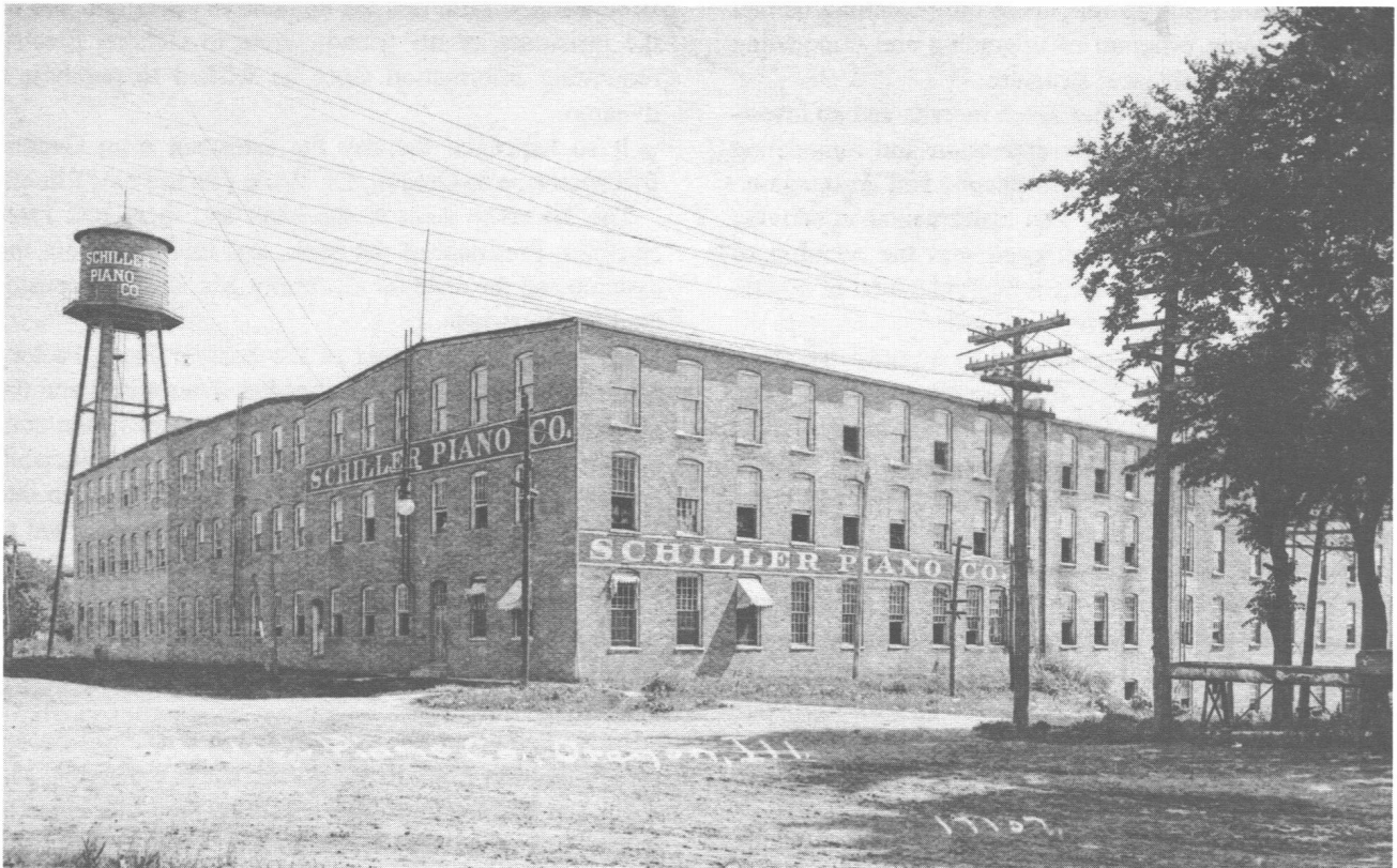
201-203-205 North Third Street
