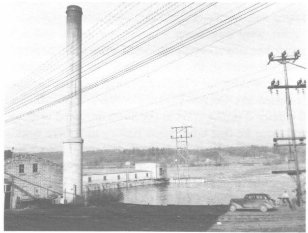
Oregon Power Plant razed some years back.
