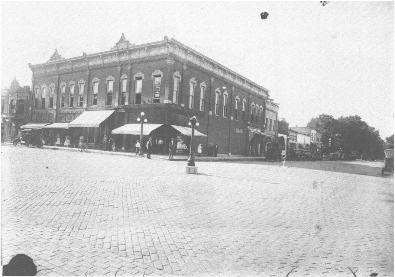
Jacobs Block, 400 Washington Street Taken from the southeast corner of Washington and 4th St.
