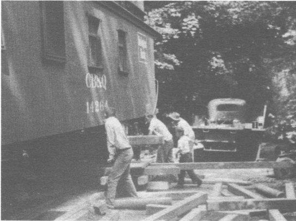
Putting wheels back under, prior to moving it. (Courtesy Charles Mongan)
