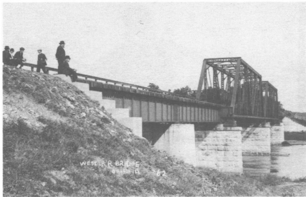
Second railroad bridge built before 1903. (Photo courtesy John Remour)
