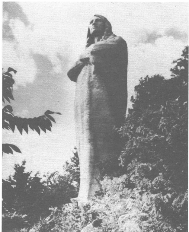
Built by Lorado Taft in 1911 as a gift to the people of the State of Illinois. Stands 48 feet high on a base 18 feet square. Contains 2,275 cubic feet of concrete reinforced with steel rods, weighs 536,770 pounds and will withstand pressure of 675,785 wind pounds. Called by Popular Mechanics in issue of March 1911, "The World's Biggest Indian."
