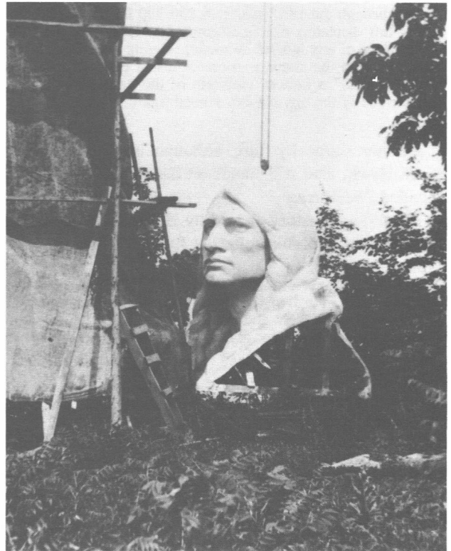
The head went up twice. This is important. It went up as a plaster model and was positioned so the piece molds could be constructed. Then it was removed and went up the final time. (Courtesy Warren Shetter)
