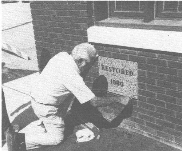
The finishing touches. (Donna Kennedy photo)
