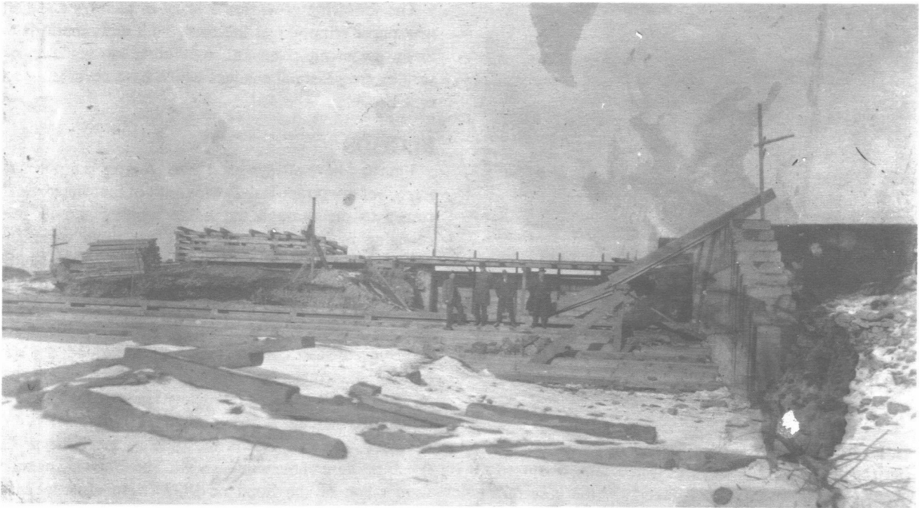
From left margin we see timbers stacked to make another crib. Then the crib itself before they push it into the water and fill it with stone. Just behind the men is a narrow gauge railroad track. The stone was brought down in little cars on this track all the way from Wooley Spring Hill quarry. Luckily it was all down hill. The right margin of the picture is the East end of the dam. Dutch Moore was drowned during the building of this dam. Robert Early wrote on the back of the photo dated March 11, 1917 that the people were: "Hossenton (engineer), Fred Hamilton (boss), Kandergarden Kid (laborer), John Miller (engineer)." Photo courtesy E. G. Landers.
