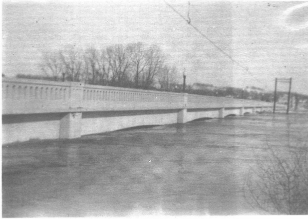
Photo by C. V. Mattison shows the bridge at Oregon at time water was up to top of arches on Monday, February 22, 1937. A drop of several feet two days later again left the ice free to pass under the arches without damage to the bridge. (Courtesy Charles Mongan)
