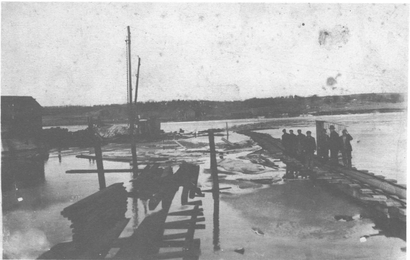
Rebuilding of the dam—1919. Noted on back of photo by Robert Early were the following names: left to right taken March 17, 1917—Bob Early (pile driver), Dick Mongan (strawboss), Bill Smith (carpenter), Ralph Bucker (laborer), Hossenton (engineer/pile driver), Fred Hamilton (quarry boss), Calvin Young (quarryman), "Woddy" Swanson (timekeeper) was not shown. (Photo courtesy E. G. Landers)
