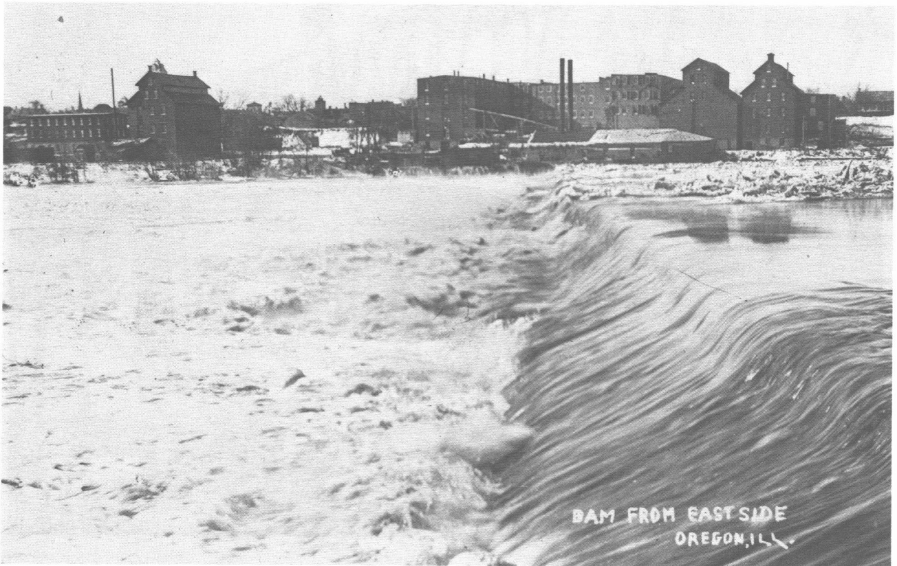
Dam from East side of Rock River.
