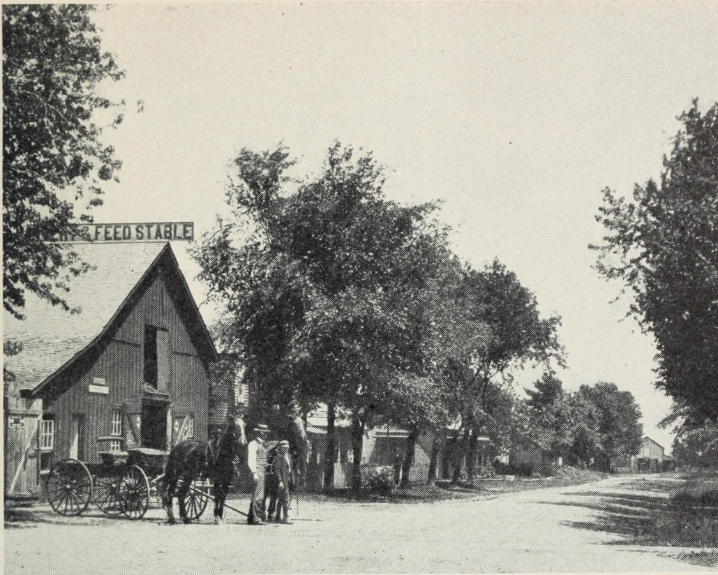
THIS OLD LANDMARK, which stood for years on the corner now occupied by the Village Hall, was torn down in April, 1906. This building was used for many years as a livery stable and was built in the fifties by Benj. and David Wagner. It passed through many ownerships over a period of fifty years, among them being H. L. Smith, Chas. Niman and Dr. A. W. Price.
