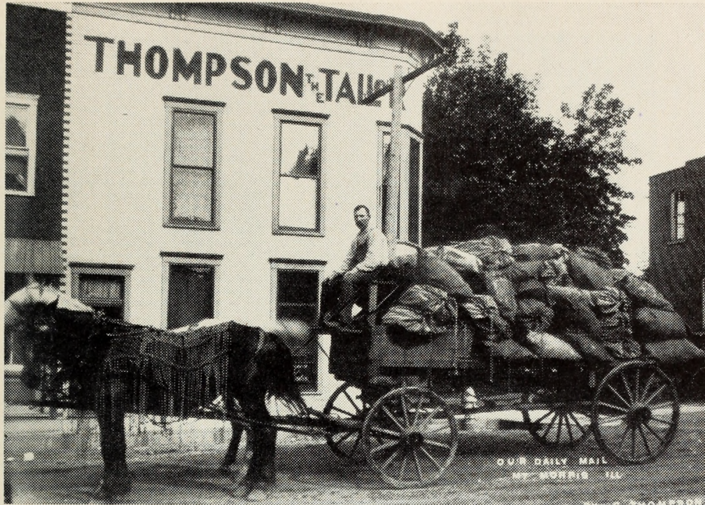
ONE OF the reasons for locating the Kable plant at the depot was the rapidly increasing volume of mail which had to be hauled to the train as shown above. Now the mail is trucked direct into mail cars which are switched into the building. Lew Lizer is the driver of the dray shown above.
