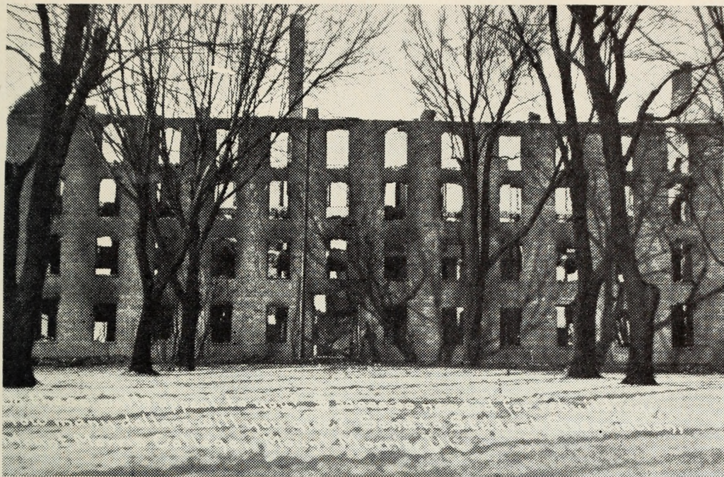
THIS IS ALL that was left of historic "Old Sandstone" after the disastrous fire of Jan. 15, 1912. The thick heavy walls were found to be solid and were used in rebuilding the structure. The new floors were made of reinforced concrete which resisted the fire of April 12, 1931.
