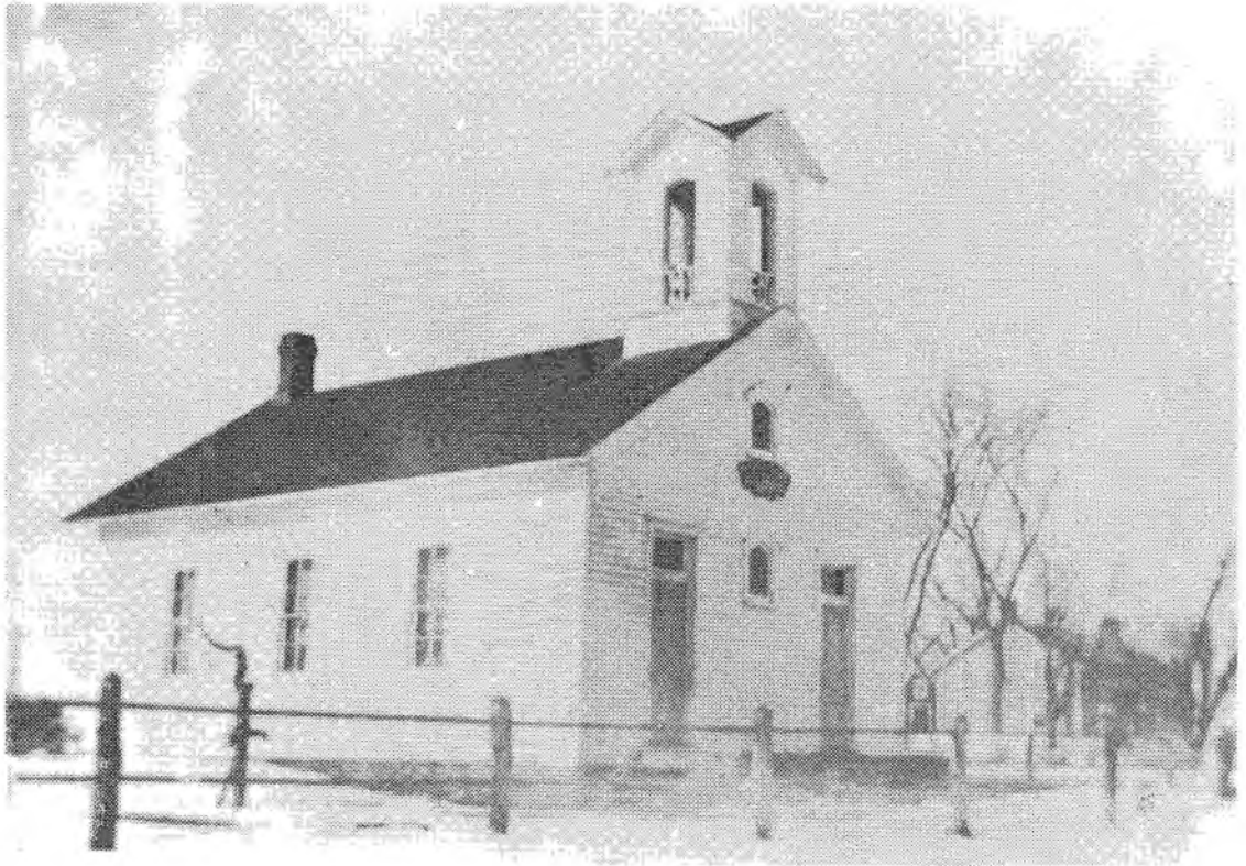
CYCLONE school Dist. 114 In 1864, the school land was in the NE corner of the Isaac Trask farm. CYCLONE enjoyed two front doors. It got its name from a cyclone that destroyed its predecessor in 1892.
