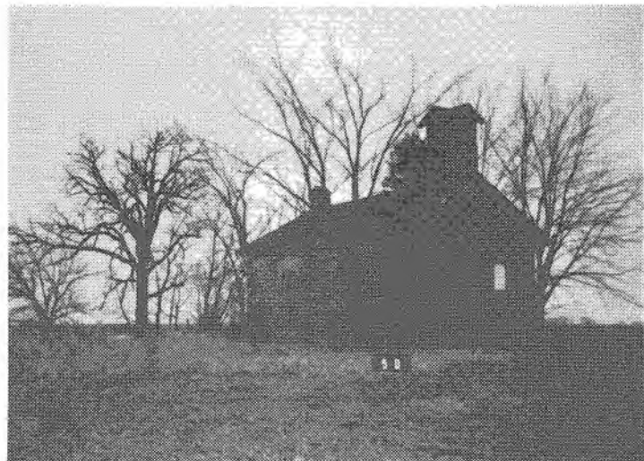
OAK RIDGE Pine Creek Twp. Dist. 50 Sec. 36 W side of Ridge Rd. & .2 mi. N of Penn Corner Rd. Building there. View N LR 1957
