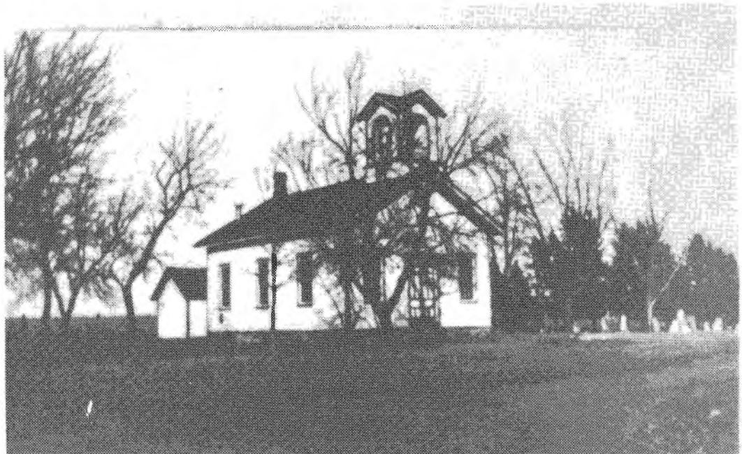
KILLBUCK school Dist. 176 In 1864, the land was a part of the A. Hill farm. This picture was taken in 1919, and the school appears to be of good construction. It stood beside a cemetery.
