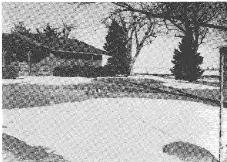
UNION CORNERS Flagg Twp. Dist. 139 Sec. 4 NW corner of Hemstock & Center Rds. int. View N Bldg. gone.
