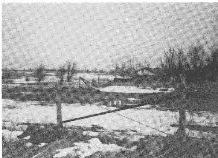
SPRING VALLEY White Rock Twp. Dist. 143 Sec. 30 NW corner of Cottonwood & Skare Rds. int. Looking NW. Bldg. gone. LR 1921.
